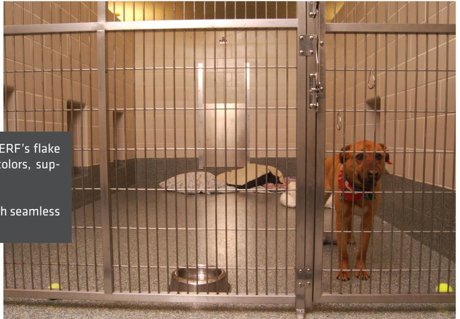
Stonhard applied a combination of Stonproof CT5, an epoxy membrane sealant, Stontec UTF and Stonglaze VSD, an epoxy wall system reinforced with an engineering fabric. These three products together produce floors and walls with enhanced mechanical strength. The flexibility of the urethane resin and the combination of Stonhard products accomplished the task of concealing the joints and maintaining a lustrous, seamless and flawless appearance.
