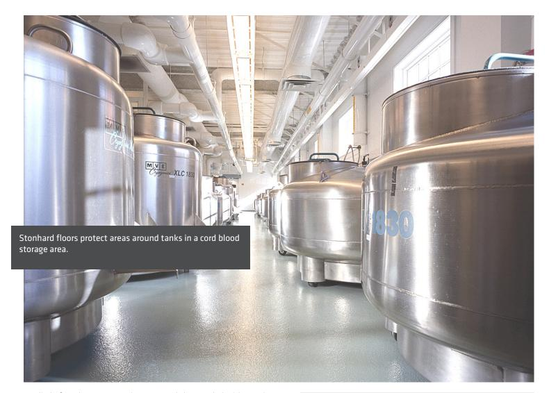
applied after the epoxy overlayment and then sealed with Stonkote GS4, a two-component, high solids epoxy coating, to further protect the floor. This coating increases chemical and abrasion resistance. The final result was a seamless, smooth, easy-to-clean, sanitary floor that would provide required protection from chemical spills and heavy, moving equipment.
