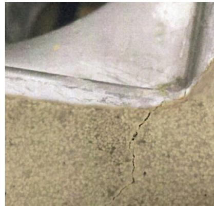
The installation of the square drain was waterproof, but cracking in the surface layer had started.
