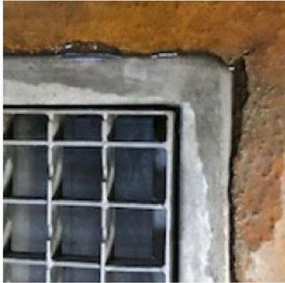
Often starting with a crack in the corner, crevices expand along the side of the drainage.
