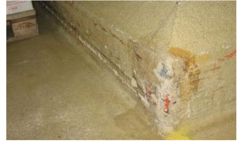
Example of concrete curb with resinous mortar. Signs of impact and damage. Concrete exposed to water will absorb and repel the covering resinous top layer and create a perfect harbor for bacterial growth.
